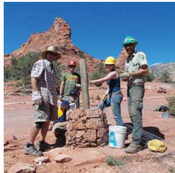
Volunteers help to install a trail sign.
